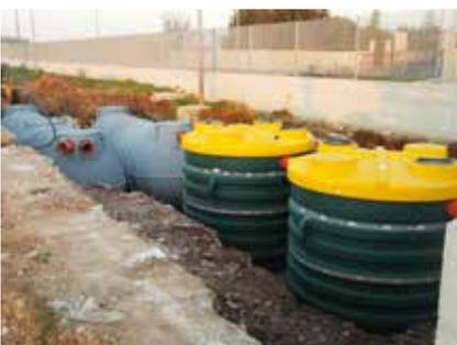
Stormwater runoff treatment (35 l/s).
